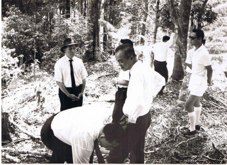
Illustration 3.7: Pow Nee observing Penang Hill's road construction
